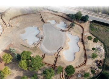
All the bunkers surrounding the greens were improved using the innovative Better Billy Bunker system. This improved layout greatly increases the drainage capacity of the surface of the bunkers, permits the water to pass through the stone at an increased rate, allows the silica sand to be kept clean and free from contamination and prevents damage from running water after heavy rainfalls.
